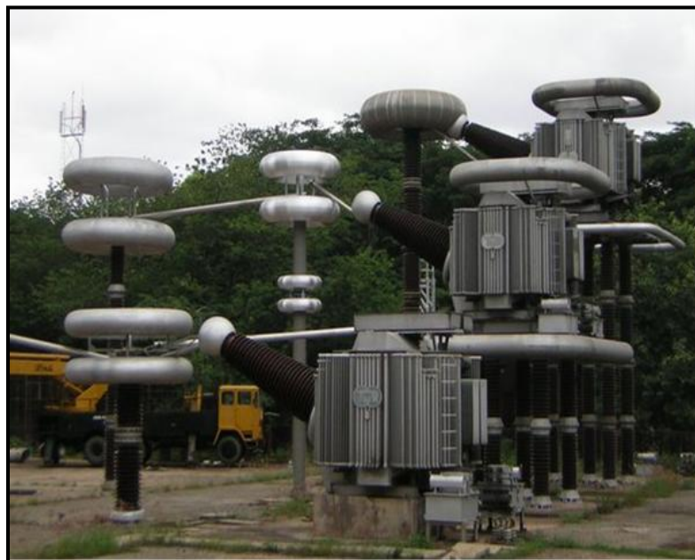
1800kV, 2000kVA Testing Transformer
