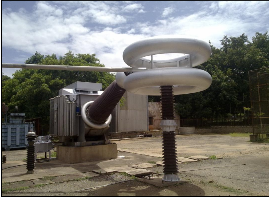
600kV, 2000kVA Testing Transformer
