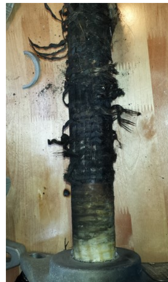
Figure 2 - Failed arrester 21353008506 with housing removed
