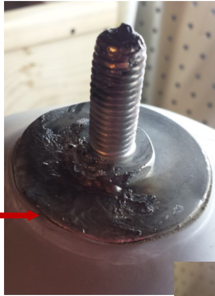
Figure 10 – Arc marks resulting from flashover on arrester 21353008505. Arrow points to area of compromised seal.
