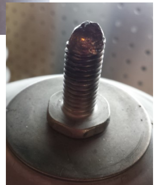
Figure 11 – Arc marks on top stud of arrester 2135008504.
