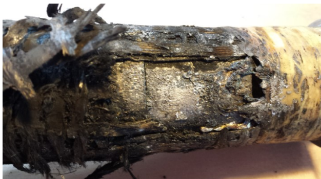
Figure 7 – Main expulsion point of failed arrester module
