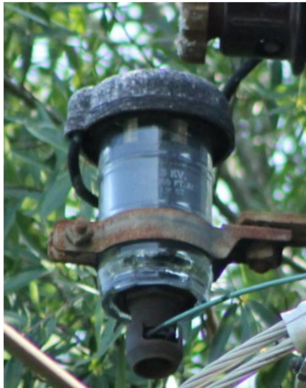
Figure 6: 1950ish Silicon Carbide Arrester in Service in 2015
