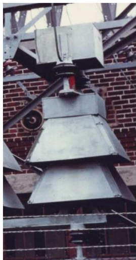
Figure 4: Oxide Film Arrester in Service in 1969
