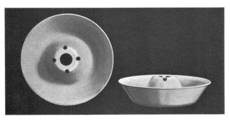
FIG. 2-DETAIL VIEWS OF ALUMINUM TRAYS USED IN THE ELECTROLYTIC ARRESTER
