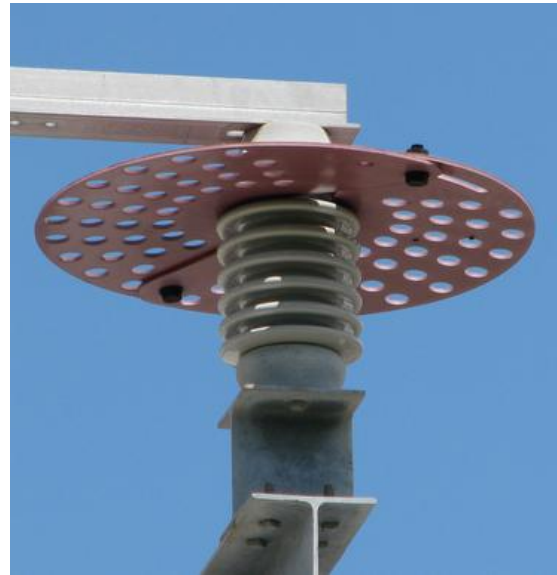
Figure 9 Barrier type wildlife protective device mounted too close to the top terminal of the insulator
