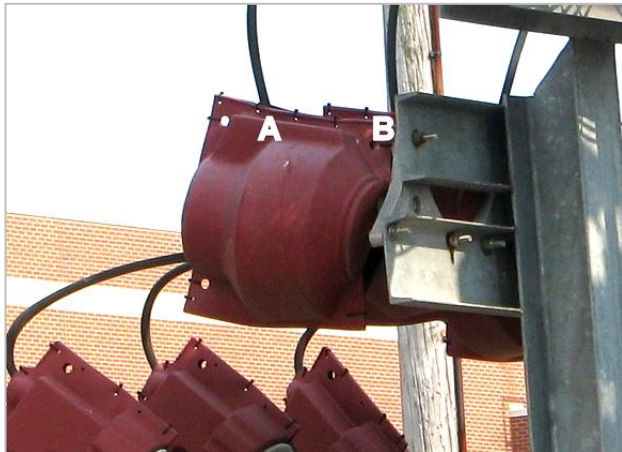
Figure 7 Example of poor lead management
