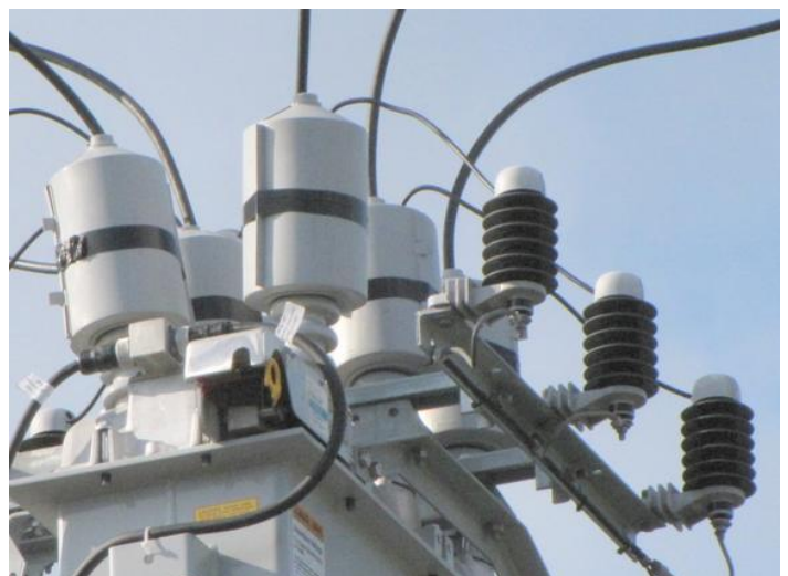
Figure 3: Cover Type Wildlife Protective Devices on Duke Power system.
