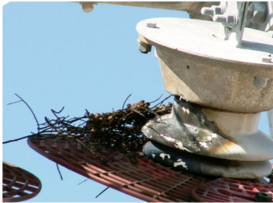
Figure 10 Barrier type wildlife protective device compromised by a bird nest
