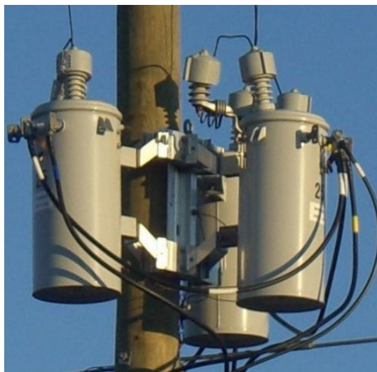
Figure 3 Cover Type WPDs on Duke Power Systems
