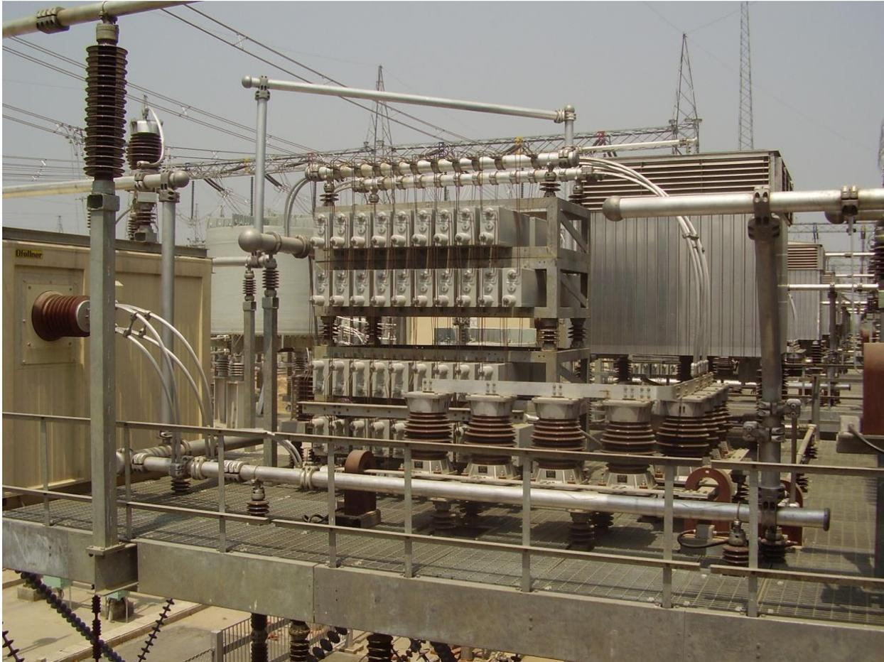
**Figure 2:** Close up of one Segment of a Series Capacitor Bank Installation. Shown are the MOV units in the front, the triggered gap in the box in the back right, and capacitors to the left of the triggered gap.
