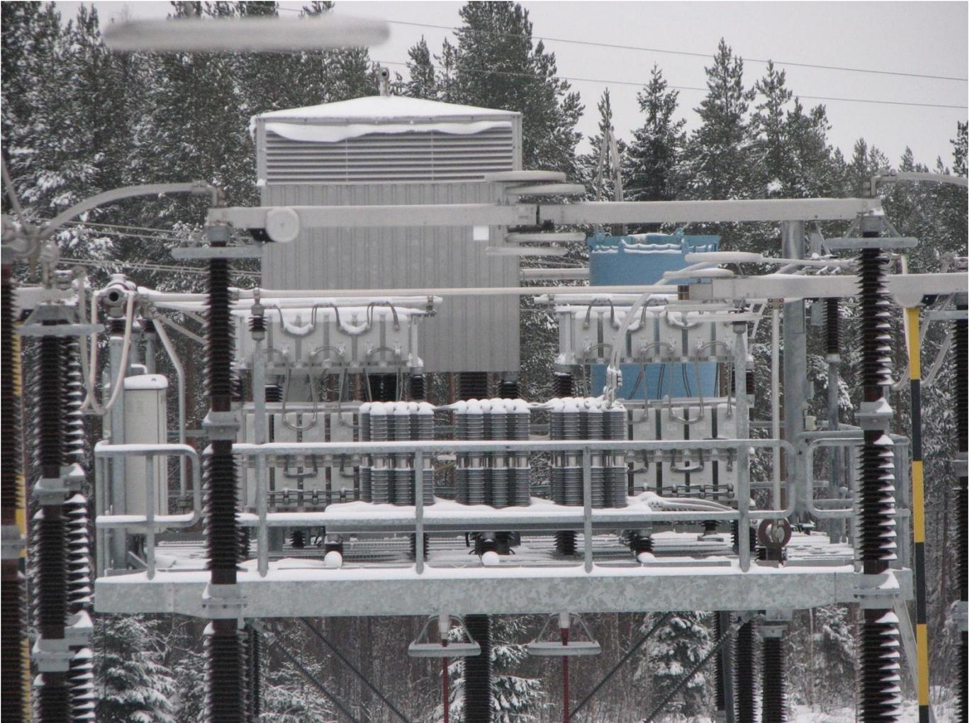
Figure 10: A Series Capacitor Bank with MOV Protection in a cold climate
