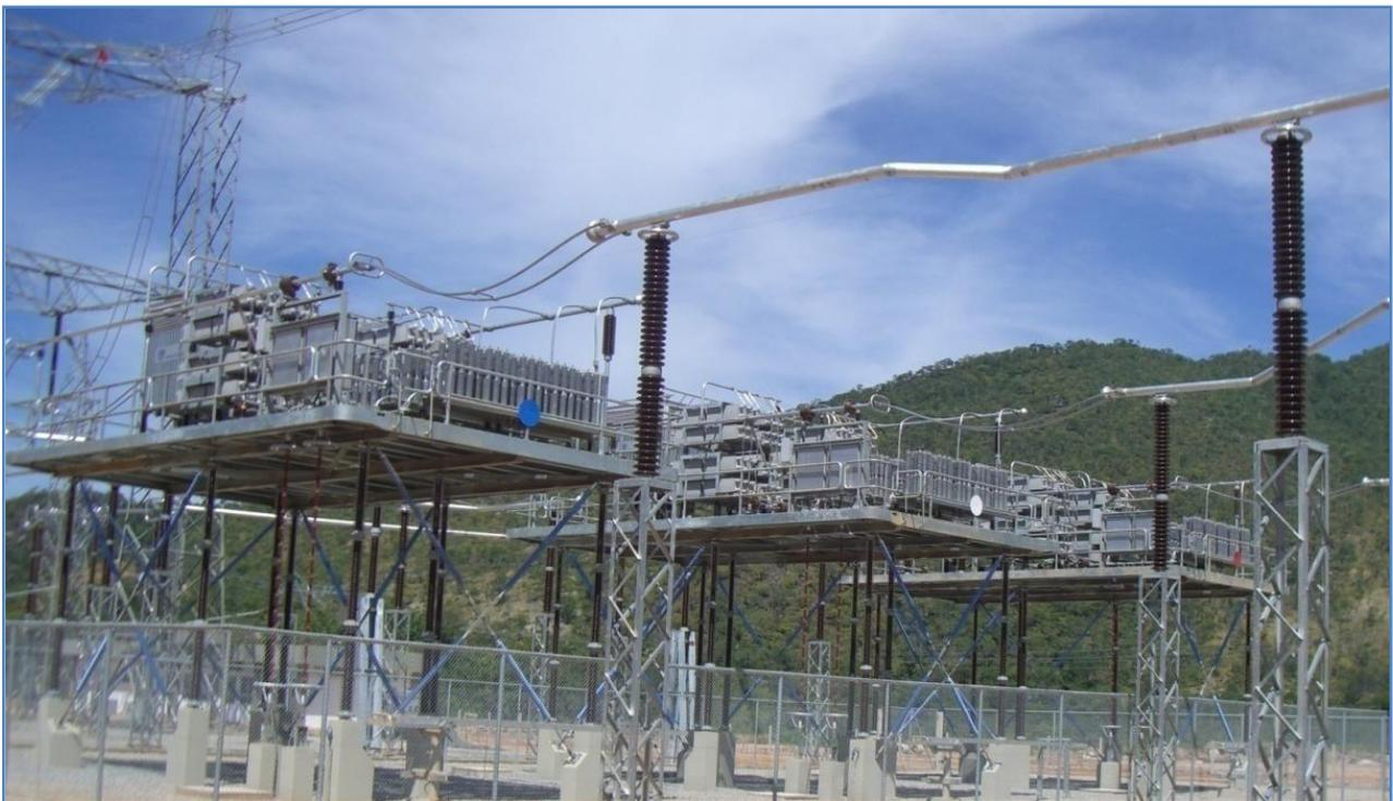
Figure 1 New series capacitor bank showing all three phases on 500kV platforms in Brazil
