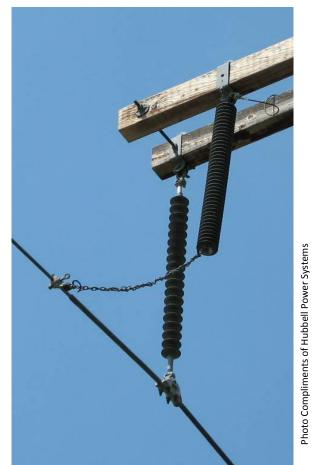
Figure 7 Lead Reinforcement with a chain
