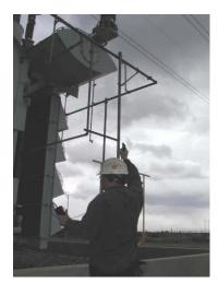
This is referred to as acoustic since this method uses acoustic transducers to detect and amplify the sound of the corona and then converted it to a more suitable audio range for the human ear. Transducers are available to listen to partial discharge within a transformer that has a grounded tank, but this method does not work on arresters unless they are of the GIS or liquid immersed type.
